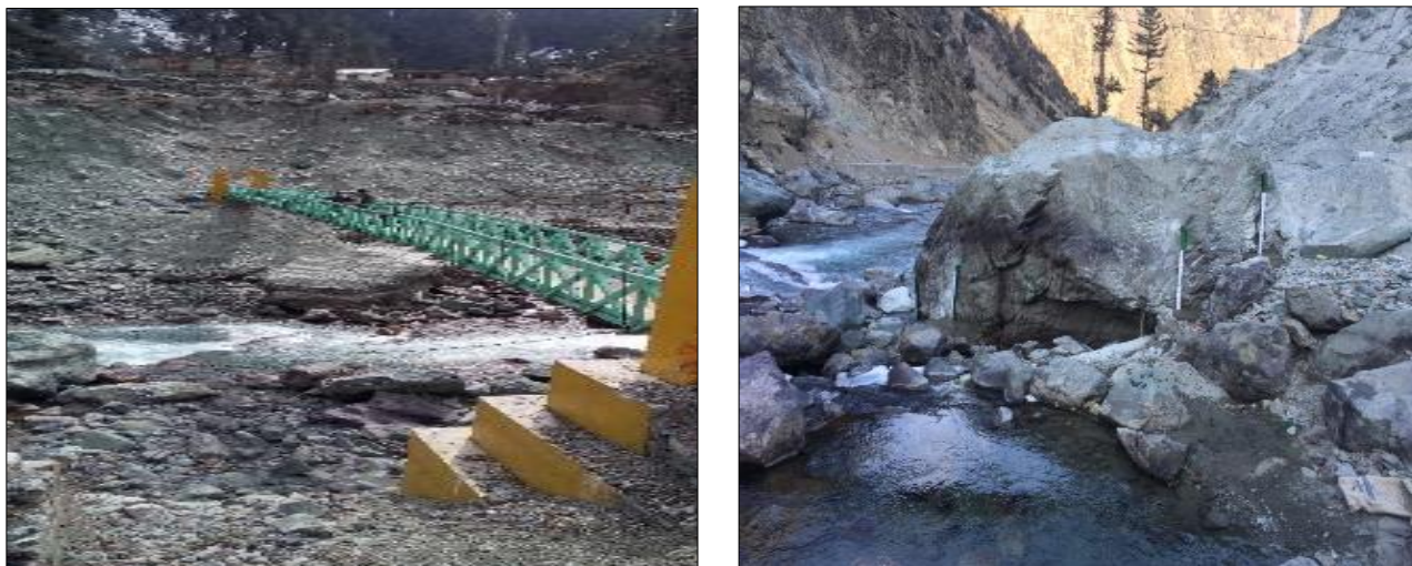
Figure 4: Gauging Station at Gabral River (Wuch Bridge)
